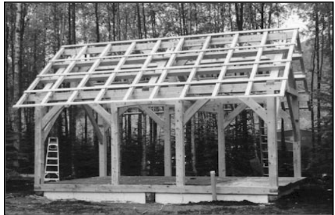
The new timber-frame "pavillion" at Discovery Cabins
