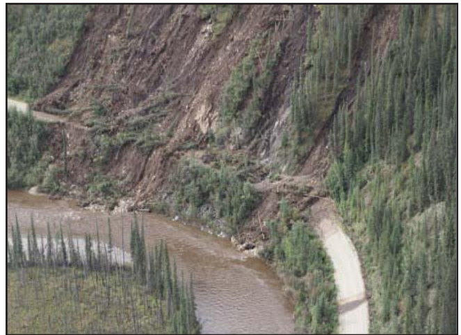
One of the "slides" --already a tenuous road connection
